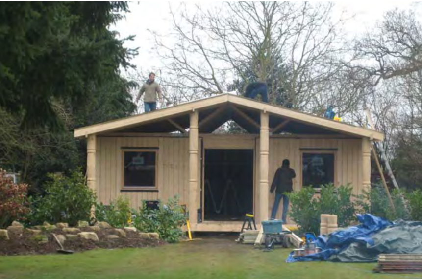
The Norwegian log cabin took just three weeks to construct
